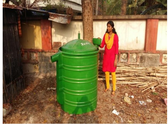
Installation of Kitchen waste processing unit nearby Canteen of main campus of Calicut, CMFRI for biogas generation for cooking on 31.10.16
