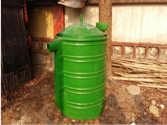
Installation of Kitchen waste processing unit nearby Canteen of main campus of Calicut, CMFRI for biogas generation for cooking on 31.10.16
